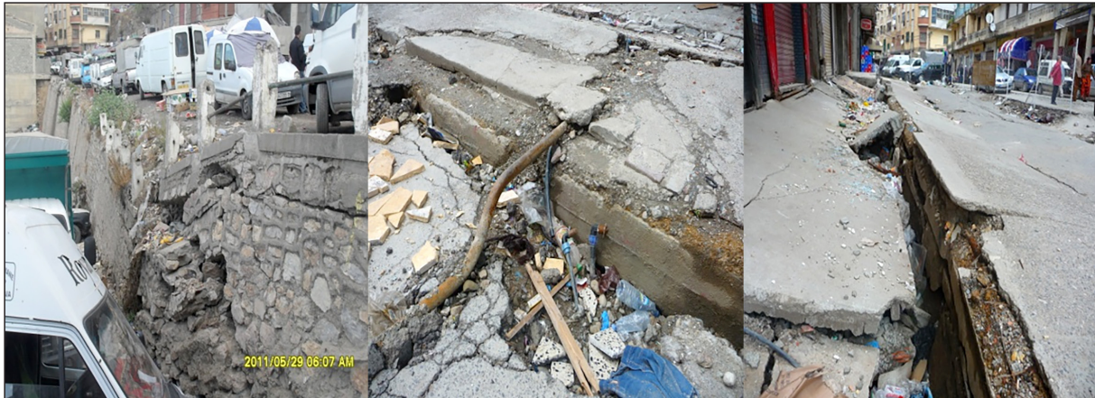
Figure 3. Dislocation of a retaining wall, subsidence of sidewalks, and cracks in pavements affecting pipeline networks.
