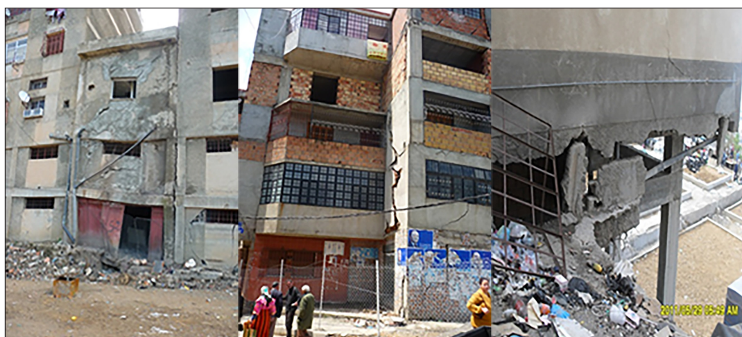
Figure 2. Obstructions observed in buildings.
