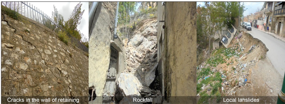
Figure 5. New instabilities registered in 2016.
